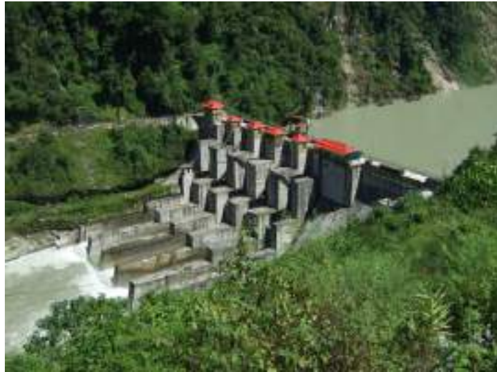
Teesta-V hydropower project
