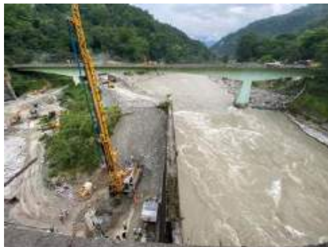
Teesta-VI Hydropower Project
